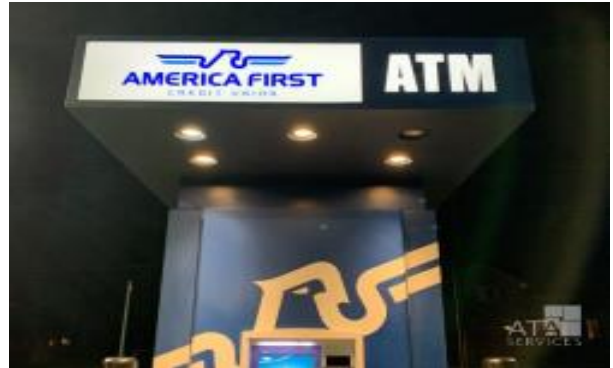
NON WORKING CANOPY LIGHT AREA
